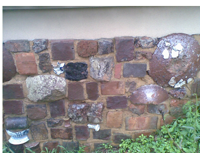
Photo author's own: A reconstructed kiln chamber walls by integrating tombai red clay from damaged noborigamas with recycled kiln materials (porcelain stands and saggars)
